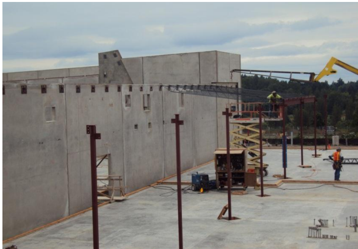
BMF Bldg. – Structural Steel & Joist Erection
