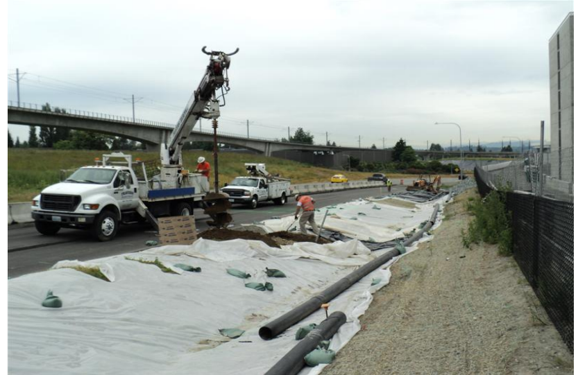
ORI: Light Pole Foundation Augering at SR 518
